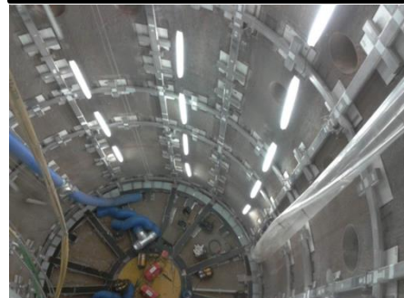
Preparation for pool liner setting-up
