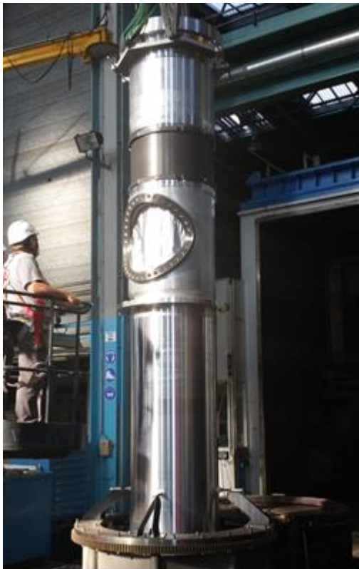
Last welding on the vessel Electron beam welding
