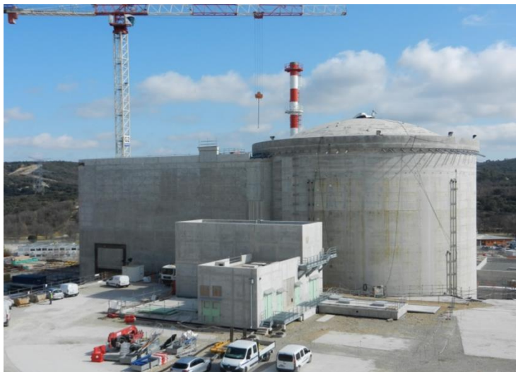
Civil work of Reactor Building and Auxiliary Unit Building nearly completed
