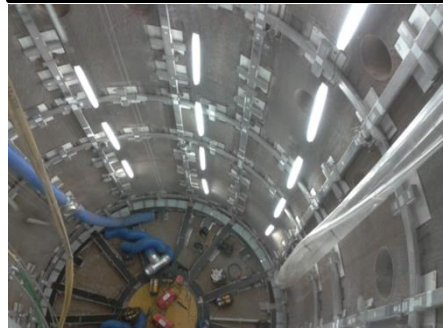
Preparation for pool liner setting-up
