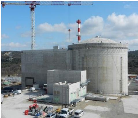
JHR Building site- Mid 2017
