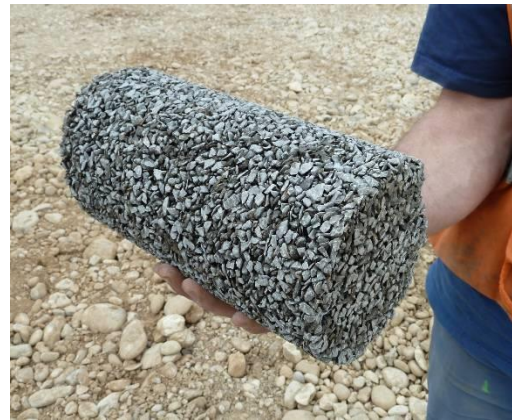
(b) Sample of the 4/6 mm crushed material injected for drainage of facing
