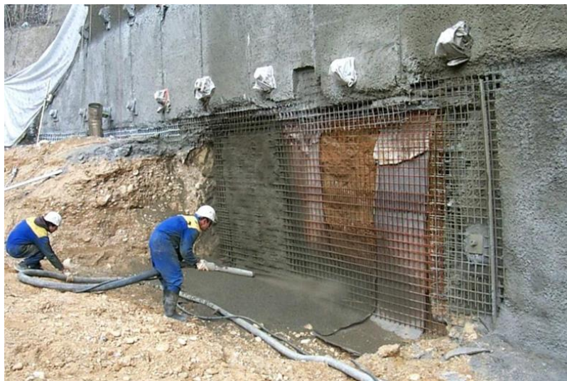
Figure 10. Construction of the facing for one excavation stage using shotcrete
