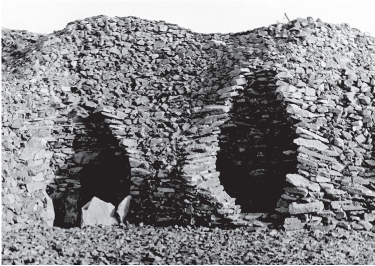
Fig.5. Small and large stones: internal arrangements - corbeling in chambers C and D (A) and survey in elevation view of the chamber and the first part of the corridor of chamber G (B) in the large cairn of Barnenez. A/Photo taken during excavations by P.-R. Giot, Archives of the Archaeosciences laboratory - UMR 6566. B/ Survey in elevation view by F. Cousseau (2016): the color of the stones is as close to reality as possible.
