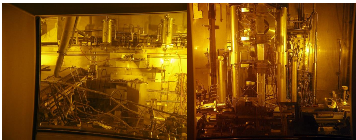
Figure 4. View of Hot Cells 418 and 421 (initial situation)
