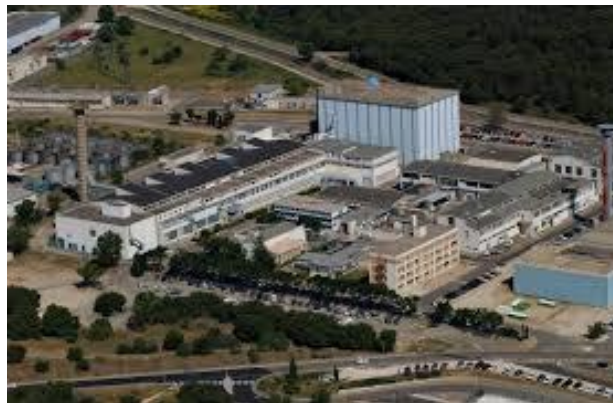
Figure 1. General view of APM
