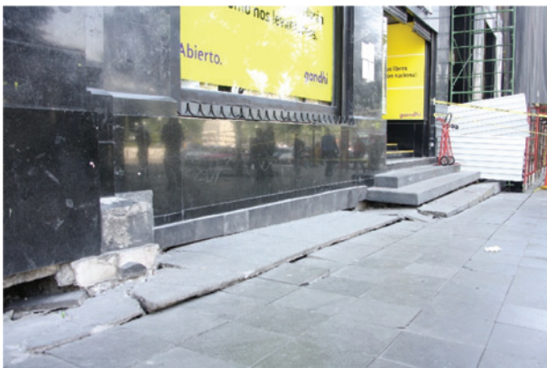
Figure 9: Evidence of soil-structure interaction in Mexico City (Photo courtesy of S. Brûlé and A.F.P.S. [69]).
