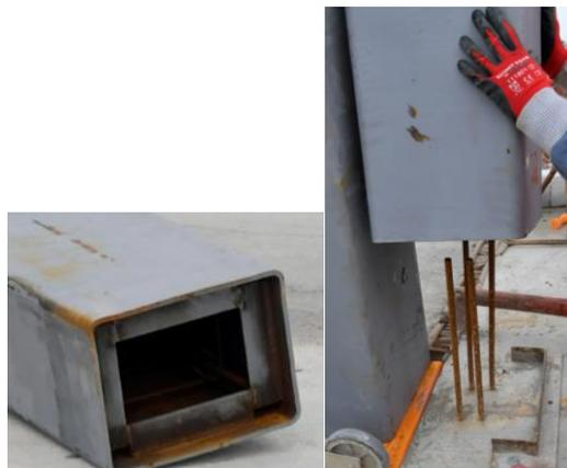
Fig. 36. Column shoe connection
