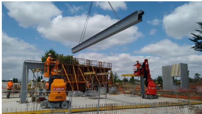
Fig. 37. Erection of the steel portal frame
