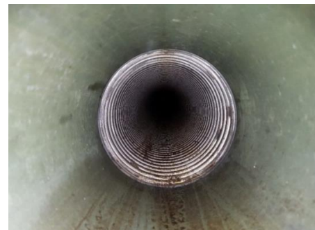
Figure 1 – View of the inside of the tested rough bore flexible pipe
