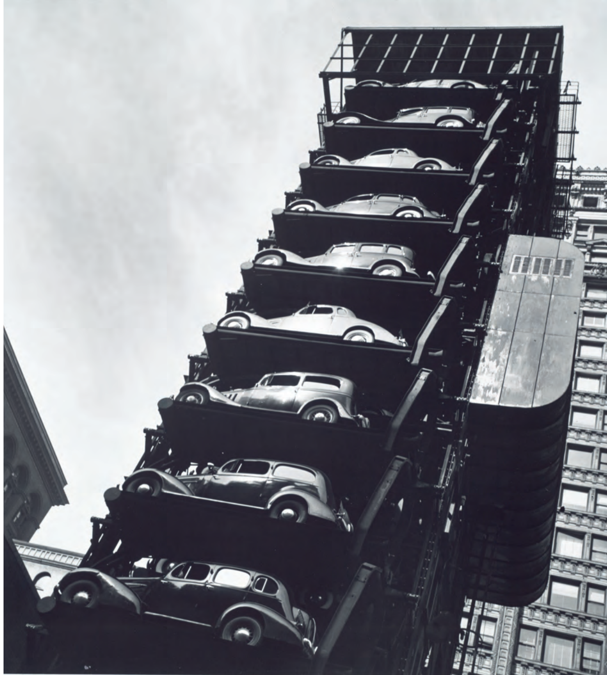
Elevator Garage, Chicago, 1936. Photograph by John Gutmann
