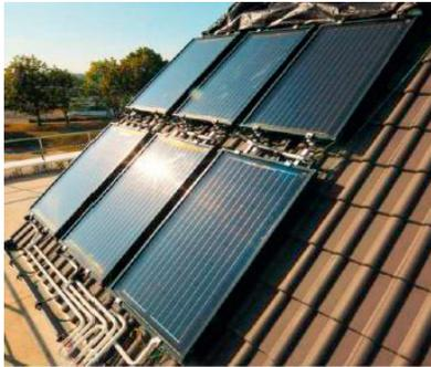
Fig.4 : Photos of the PV-T modules installed on the roof of BESTLAB
