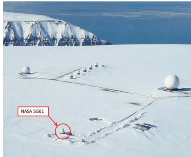
Figure 1. Aerial photograph of the Svalbard NEN site showing the location of SG61.
