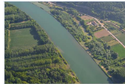
Channel restoration scheme
