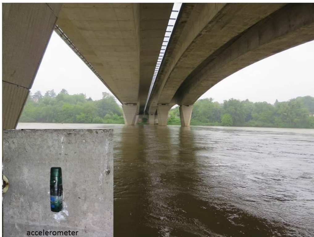
Figure 4. .View of the site in April 2019 and zoom on the accelerometer.
