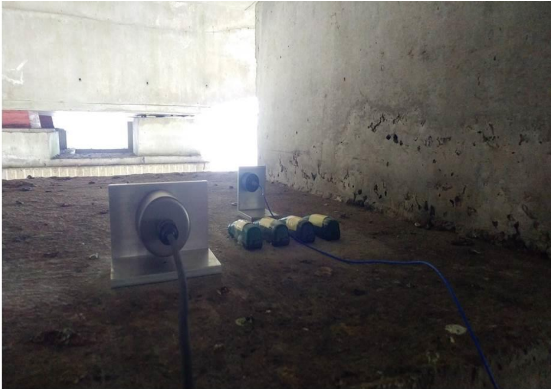
Figure 5. Accelerometers on the real bridge.
