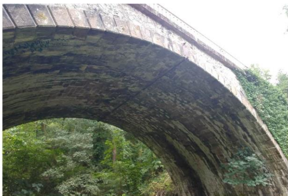
a) view of the bridge masonry
