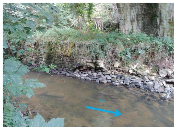
b) flow and abutment scour
