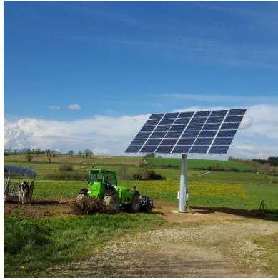
Agricultural exploitation using solar tracker Credit: GAEC du Faisan
