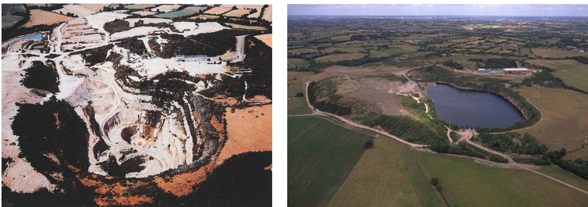
89 Figure 2: Aerial photographs of the La Commanderie site: a) at the end of the period of 90 mining operations; and b) after the first rehabilitation (AREVA, 2013; Chapot et al. , 2010)
