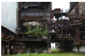
Hauts-fourneaux U4 Uckange, Lorraine, 2014
