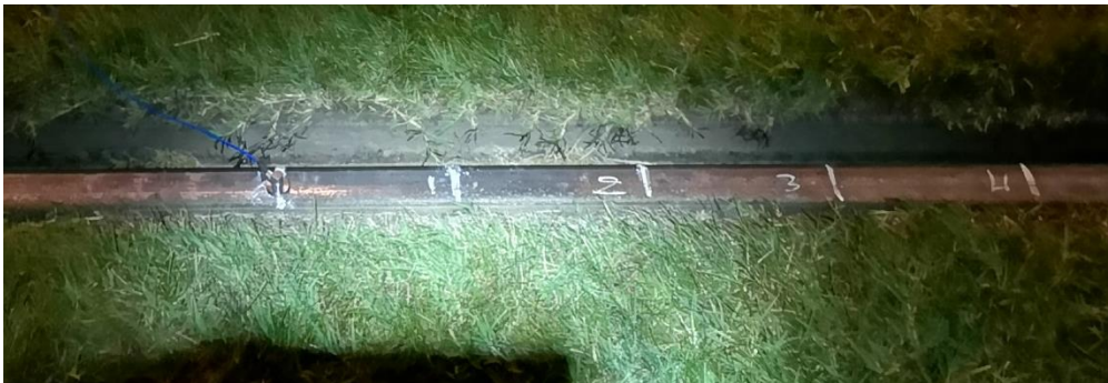
Figure 8: Accelerometer fixed on the embedded rail with first impact location marks for the measurement of the vertical decay rate according to EN 15461 (track B)
