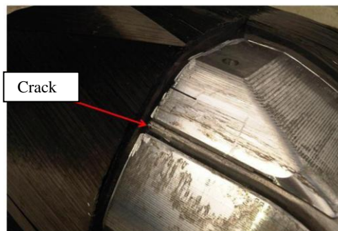
Figure 10. Crack on the welded joint - source of the leakage
