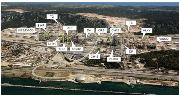
Figure 1 : Locations of different exhaust stack in the refinery. Main aerosols exhaust stack are the boiler CH11 and flare T2.
