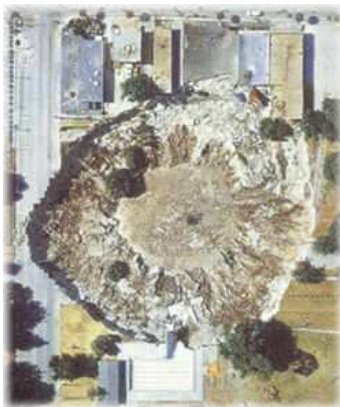
Fig. 1. Land Subsidence (sinkhole) in Central Kansas related to Salt dissolution (after USGS water science).
