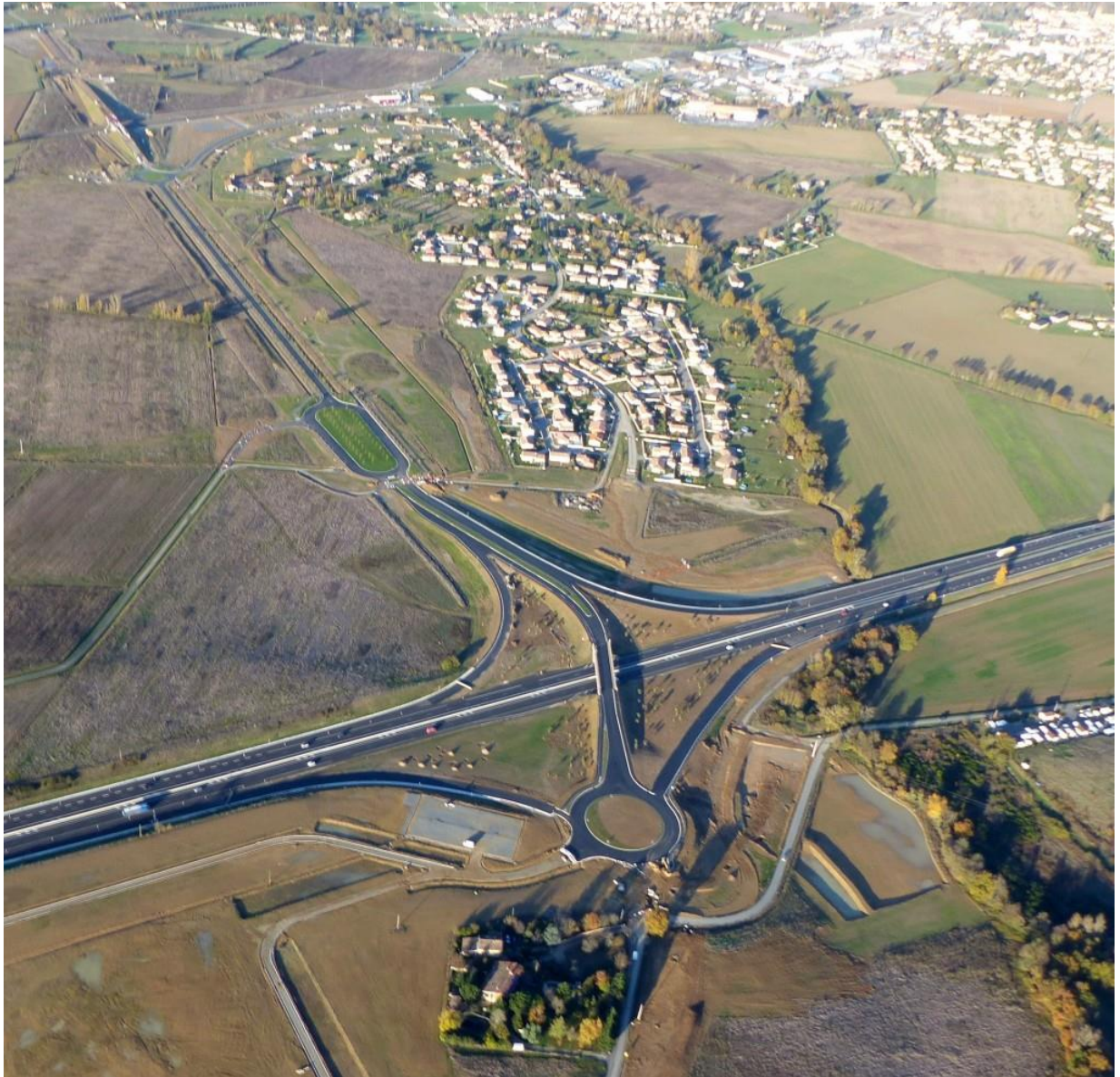
Aerial view of EIP area (east)
