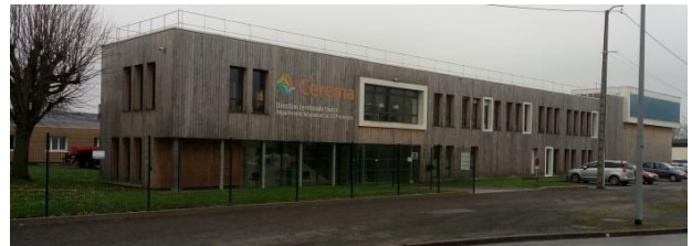
Figure 1: Picture of the case study office building
