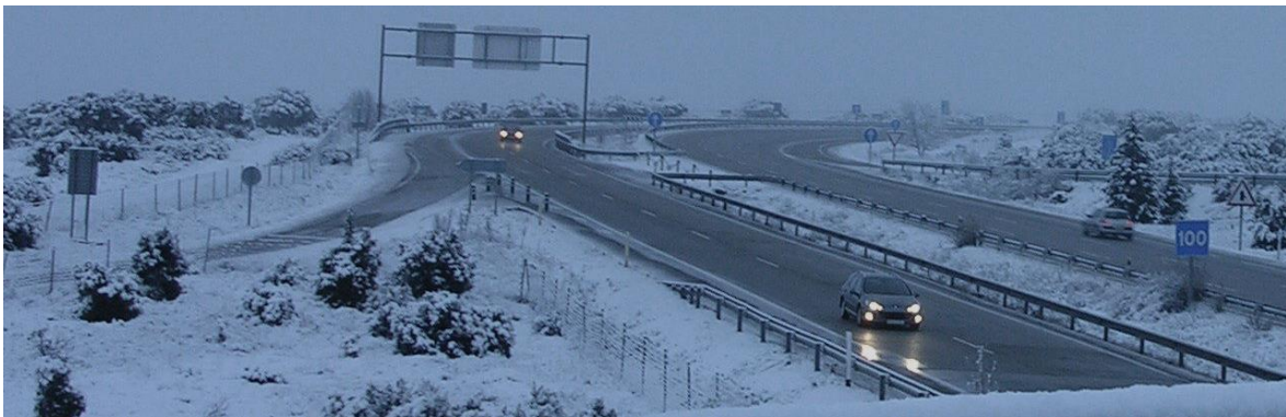
Figure 6 Section 2 – Highway A2 Spain.
