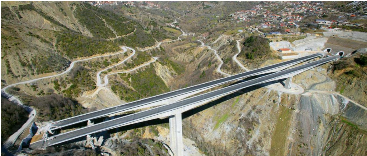
Figure 7 Metsovo bridge. Egnatia Motorway.
