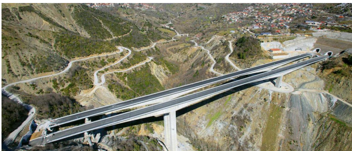
Figure 7 Metsovo bridge. Egnatia Motorway.
