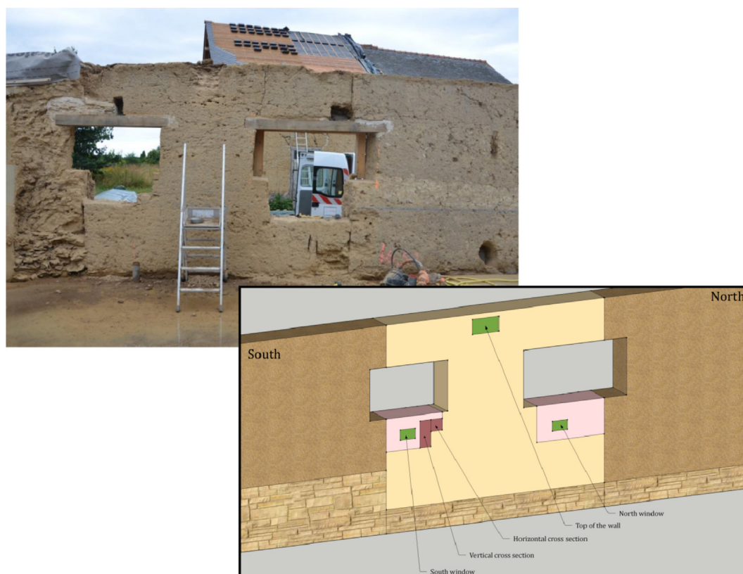
Fig. 2 View of the three different construction stages (North, middle and South) identified in the wall, seen from the inside of the building. Sampling concerned the middle stage (yellow): pink parts were collected, with particular samples for thin sections (red) and material identification (green).
