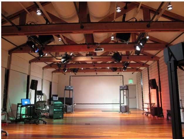
Figure 8. The Stage in 2011, 16 speakers in 8 + 8 configuration, 8 subwoofers in the bottom of the main towers
