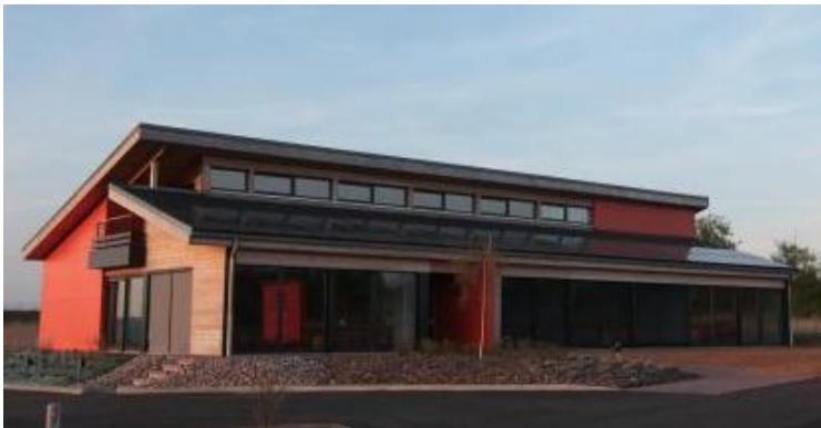
Fig. 1 View of the south facade of the case study building
