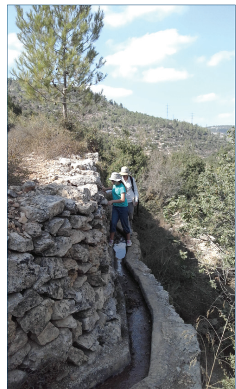
Traditional open air channel leading spring water to a field
