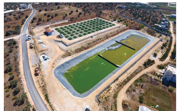
Missilya wastewater treatment plant
