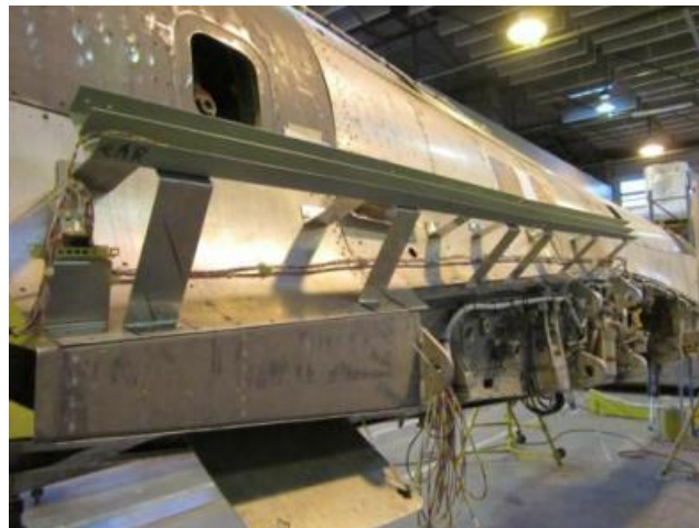
Figure 10 : Raceway general installation view
