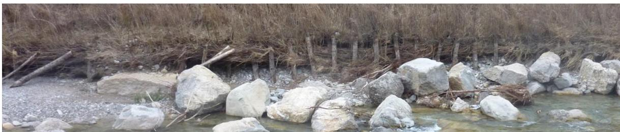
Figure 11: Fascine protected by one row of large riprap, destroyed on the Büech River after a 10-year return period flood involving local scouring of about 1 m. (picture courtesy of G. Piton).
