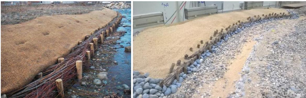
Figure 1: Fascines (a) in the field (courtesy of P. Belleudy) and (b) in the flume (example of full protection: fascine + riprap toe)
