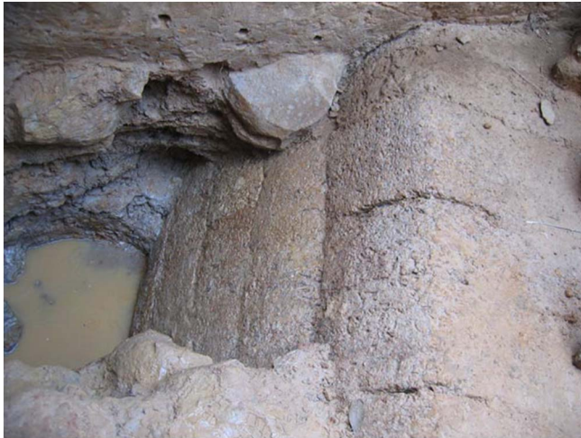
Fig. 12. Spillway at Bam Penh Reach, north of Angkor, showing ogee form at top layer of laterite. (Photo by Andrew Wilson.)
