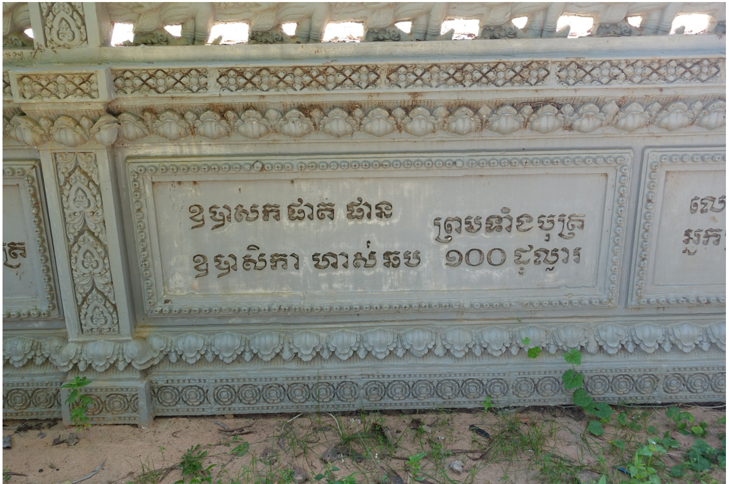
Fig 4. Contemporary Khmer pagodas list individuals who donated to the construction of the temple. This photograph was taken by Sarah Klassen.
