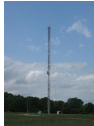
Figure 13: Picture of the instrumented mast of 60 m at Lannemezan Site
