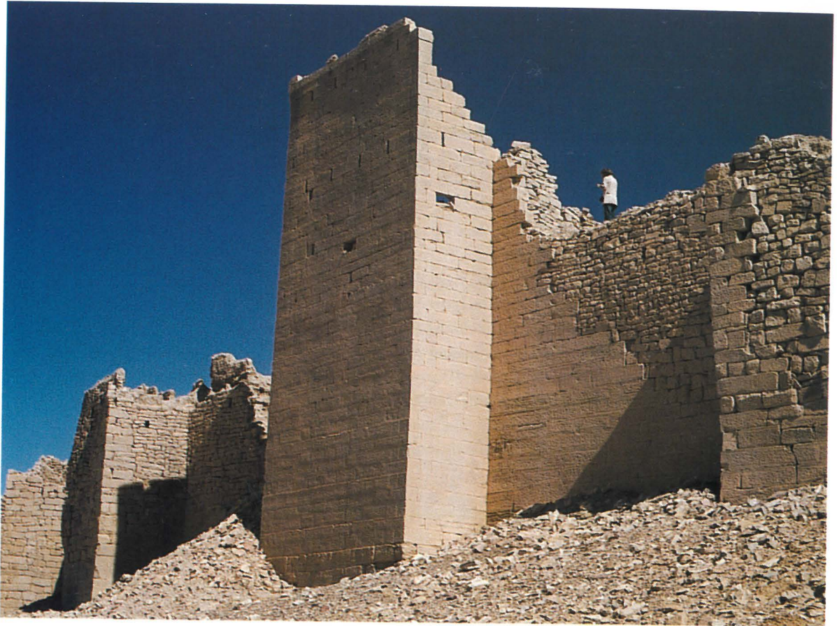
FIG. 48 The southern towers of the wall at Barāqish. (Photo: J.-F. Breton)
