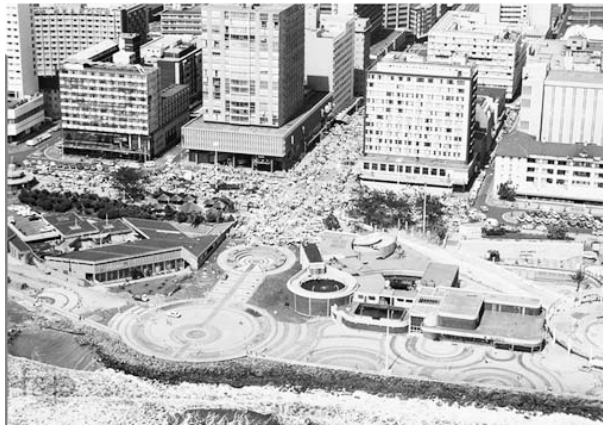
Figure 4. The 1983 upgrades implemented. The Architectural language of the implemented upgrades and the predominance of the built form of the city behind it is regionally contextualised Modernism
