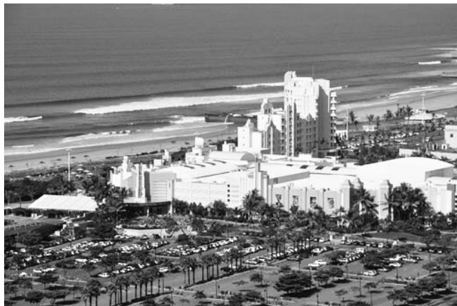
Photo 7. A view of one of the main access points to uShaka Marine World. The extensive use of thatched roofs and the inclusion of motifs derived from the isiZulu culture is applied in a rather post-modern way. Some of the components speak more of a tropical island image as there is no direct vernacular construction to accommodate the programmatic function required
