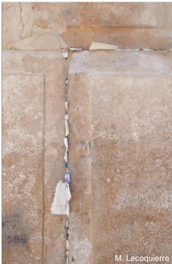
Figure 44. Notes put in the cracks of the Haram al-Ibrahimi's wall, at the location of the "seventh step". Picture taken by the author, 2018.
