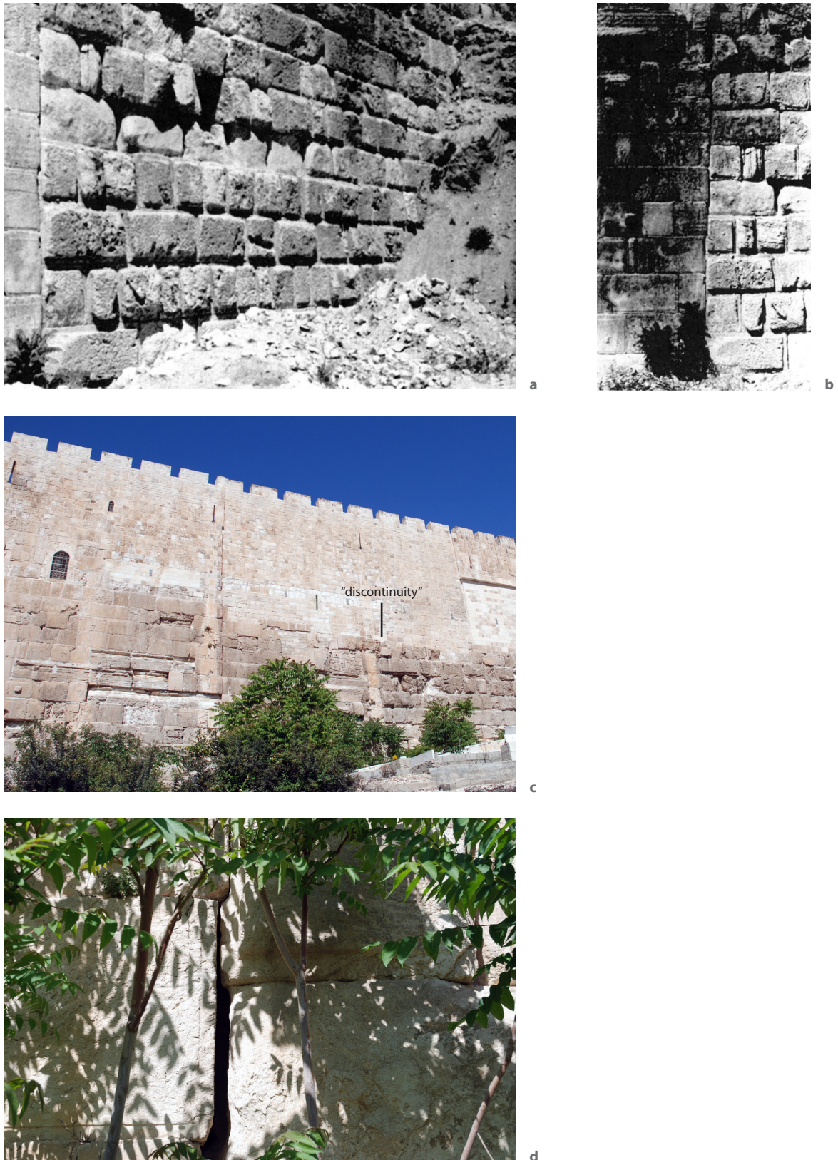
Figure 3 - Eastern wall of the Haram esh-Sharif, seen from the south-east: the "discontinuity" between the Herodian wall and another earlier section of the wall (Solomonic, Persian-era, Hasmonean?). On the left, smooth-sided stones from the Herodian part of the wall, built up against bossages from the part of the wall located to the north of the "discontinuity". a-b. The "discontinuity" as demonstrated by E.-M. Laperrousaz, 1973: fig. 3-4; c. The "discontinuity" as it is visible today, general view of the eastern wall, looking towards the south-east corner; d. The "discontinuity" as it is visible today, detail of the lower section of the currently visible part (photograph: F. Porzia).
