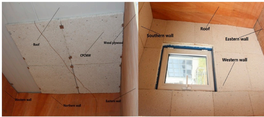
Fig. 13. cPCM wallboards installed on the ceiling and walls of the test cell [121]. Copyright (2019), with permission from Elsevier.
