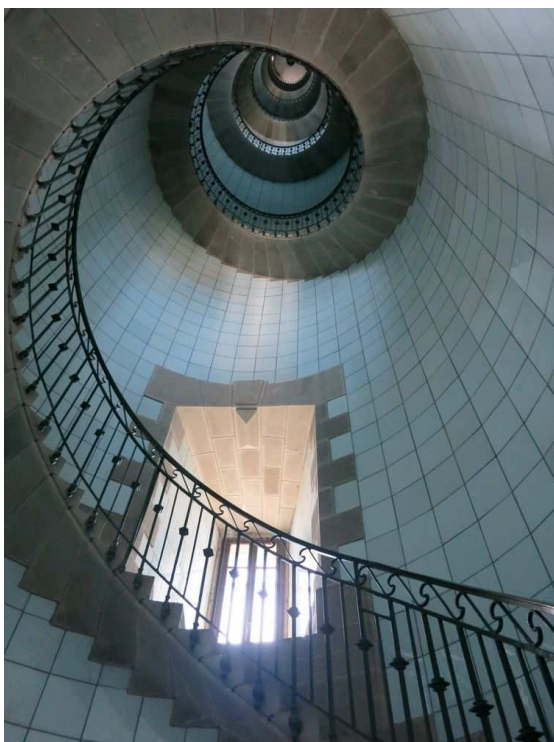
Figure 5 – Internal view of the lighthouse
