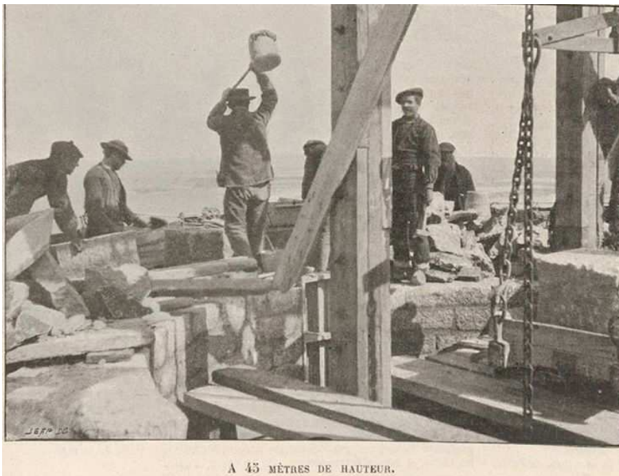
Figure 8 - Construction of the Ile Vierge lighthouse [4]
