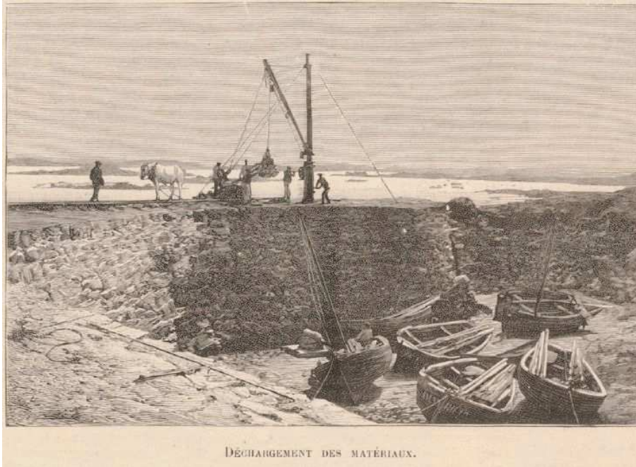
Figure 7 – Loading and unloading on the Ile Vierge [4]
