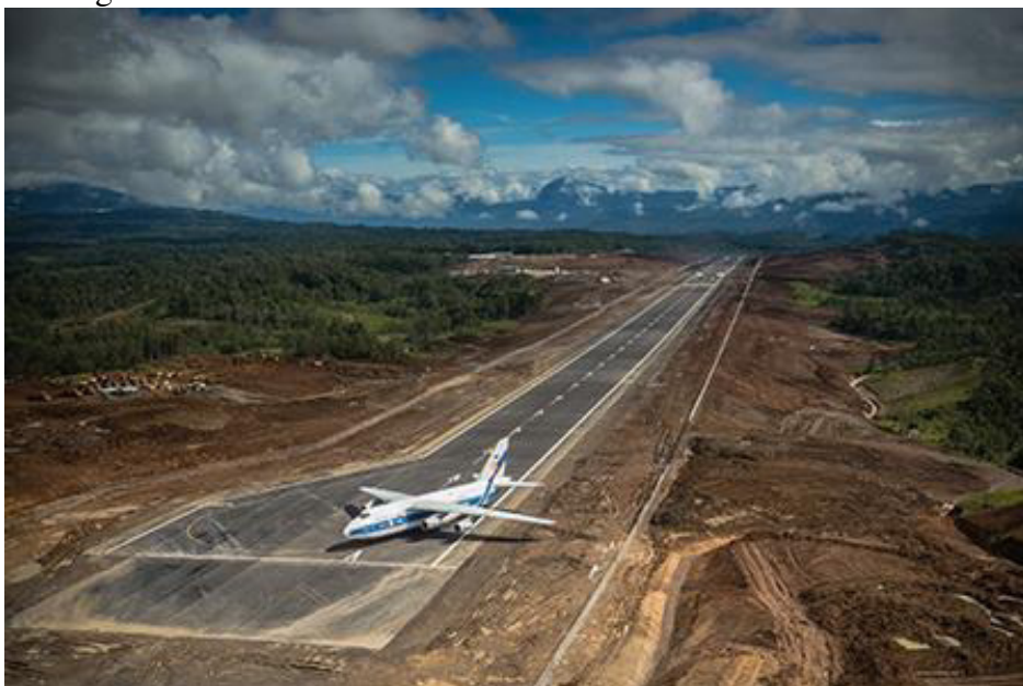
Figure 4 - Komo Airfield (Source WT Partnership website, http://wtpartnership.com.au/our-team-experience/png-lng-komo-airfield-png/ ).
