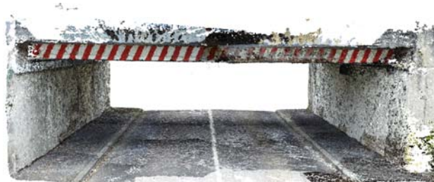
Fig. 4: Point cloud of the tunnel
