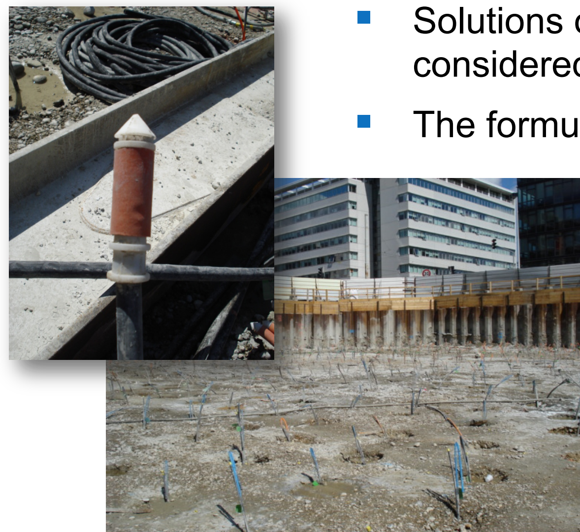
Ground stabilization on building site (Wöllner GmbH&Co.KG)
