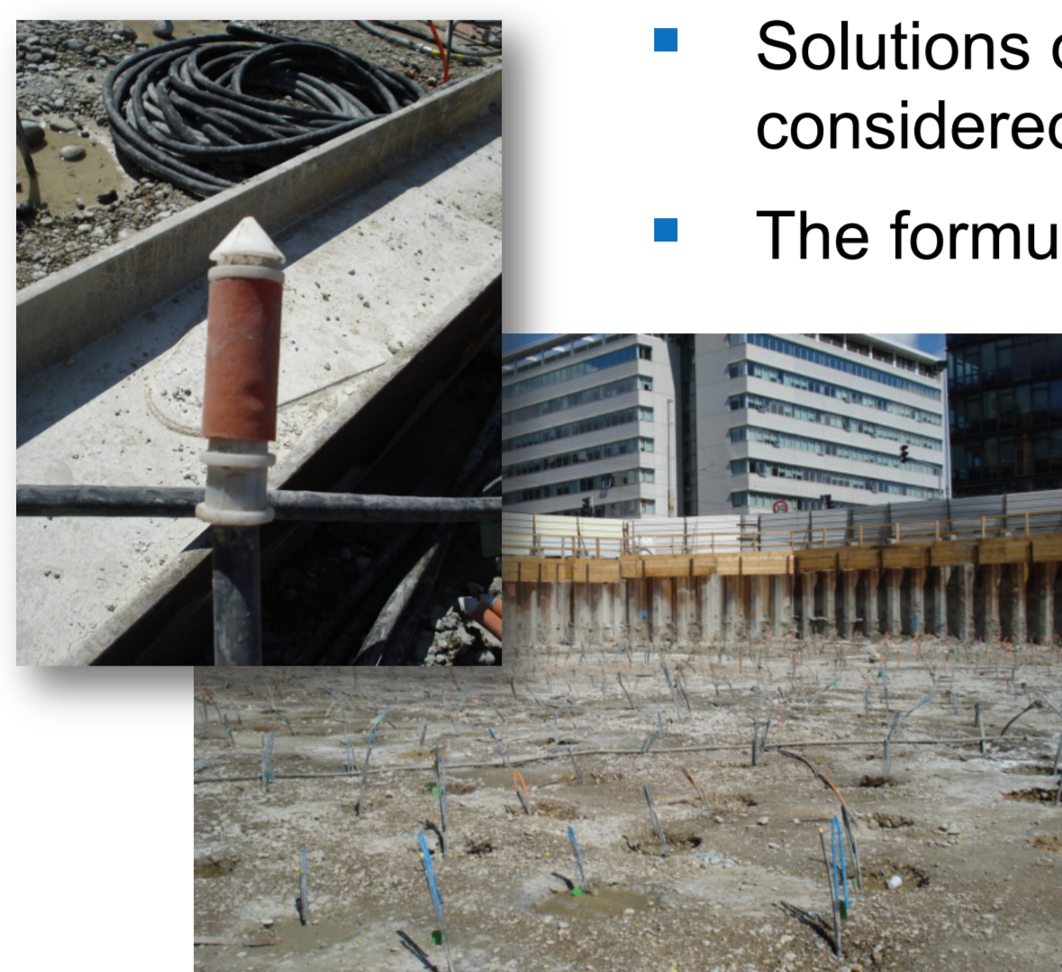
Ground stabilization on building site (Wöllner GmbH&Co.KG)
